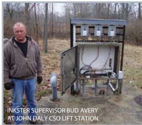
CSO LIFT STATION WITH BARNES SH SERIES
